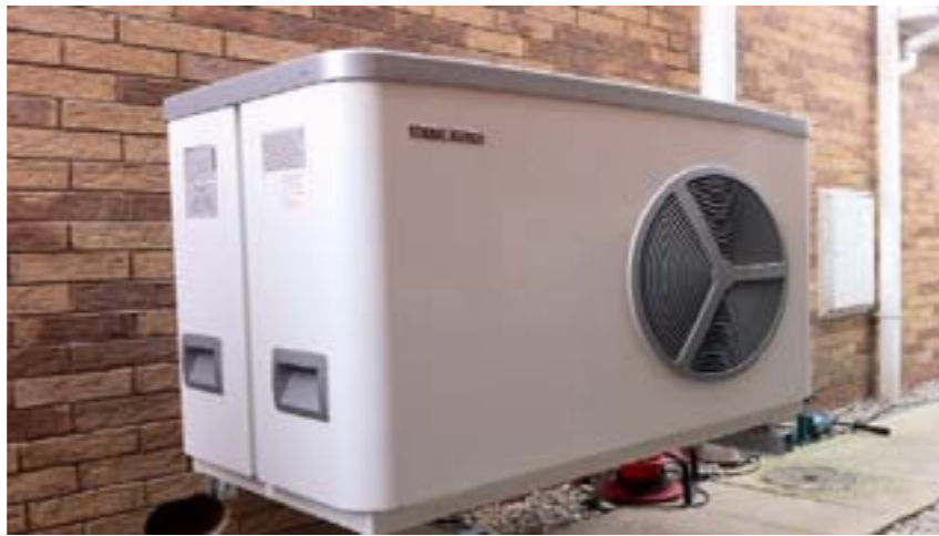
Stiebel Eltron's WPL10ACS air source heat pump is linked up outside and also provides cooling
