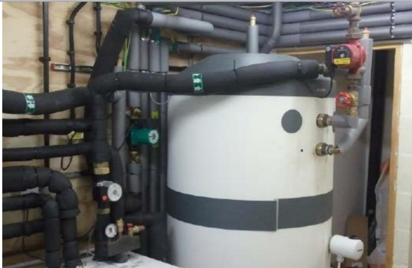
"We installed the equipment in a separate plant room, 35m away from the main house, taking heat from the farm's man made pond, via collector loops, to the ground source heat pump. A pre-installed pipe now takes heating and hot water from the plant room to the main house, to feed the under floor heating and hot water outlets.
