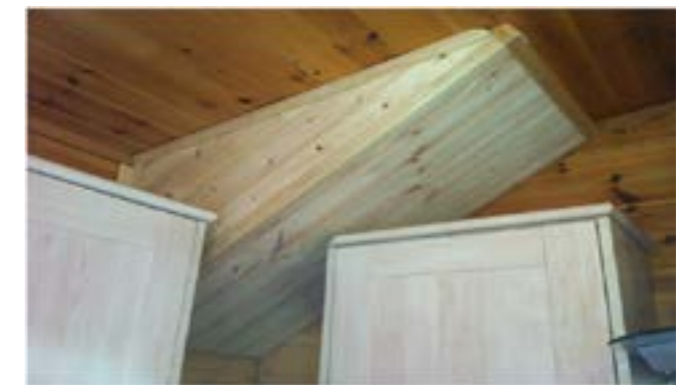
Boxed in ductwork through kitchen to loft space
