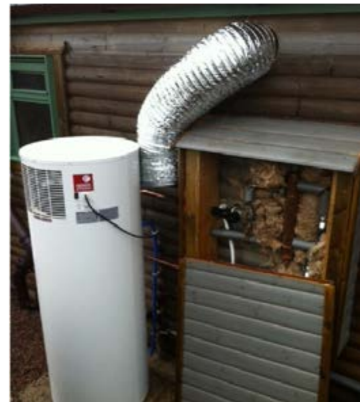
Warm air duct and WWK300 air source unit
