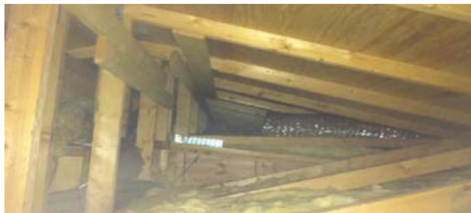
Duct sucking warm air from the loft space
