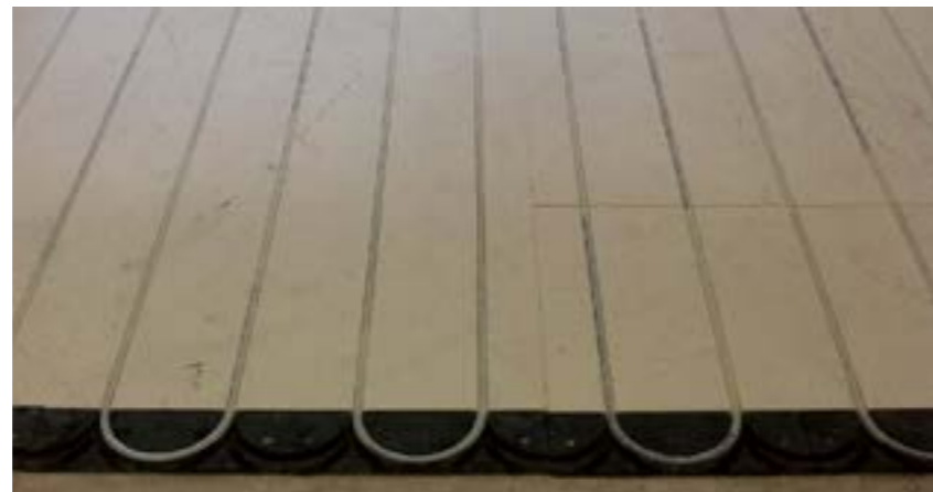
Underfloor heating has been installed on the property's ground floor
