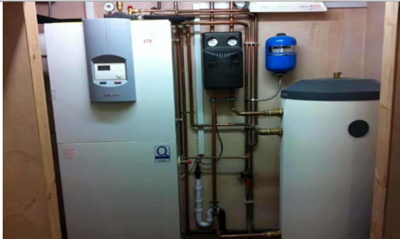
The heat pump and cylinder are discreetly positioned in a plant room
