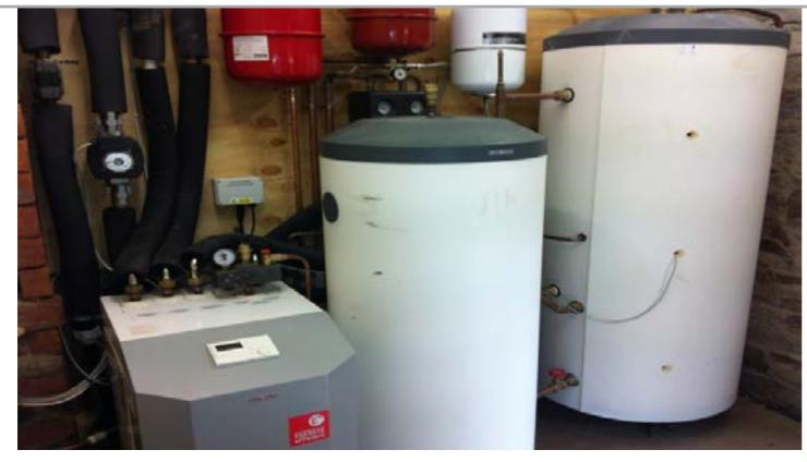
"The solution for Russian Cottage was a ground source heat pump using land available around the cottage, to install 500m of ground loop.
