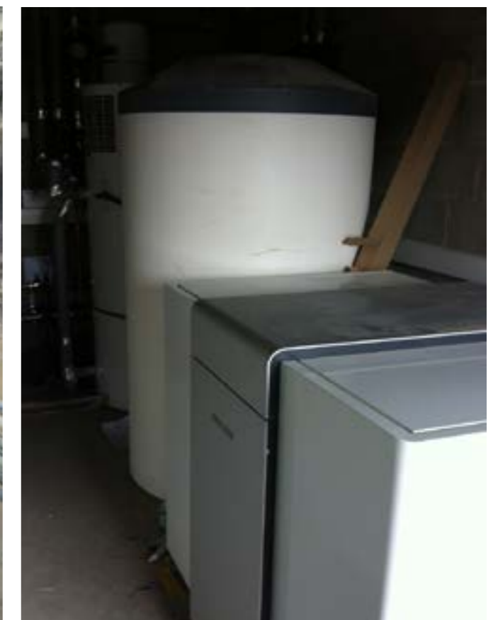
The units fit compactly into a small plant room with minimal fuss
