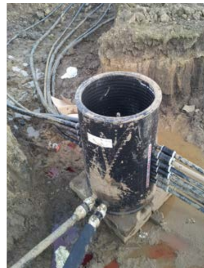
The ground source system takes advantage of outdoor space
